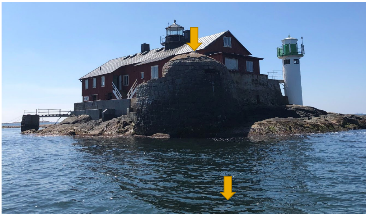
Figure 20. A ship noise measurement station deployed at the island of Böttö, Sweden, adjacent to the main fairway into the port of Gothenburg. The upper arrow indicates the position of a microphone, while the lower arrow indicates the position of a hydrophone at 13 m depth.
